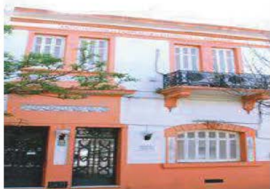
Headquarters of the National pharmacist organization (Asociación de Quimicay Farmacia del Uruguay)
